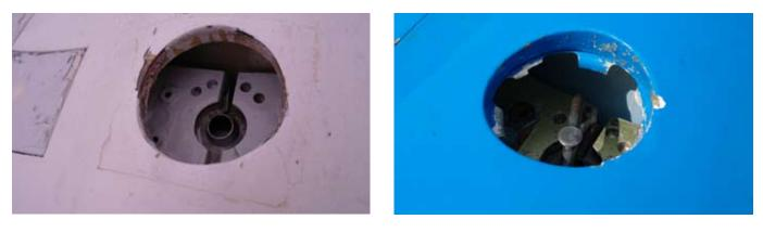
**Figure: 4 (a)** Tapered portion of bevel bolt protruding, indicating upper bevel bolt fully expanded
